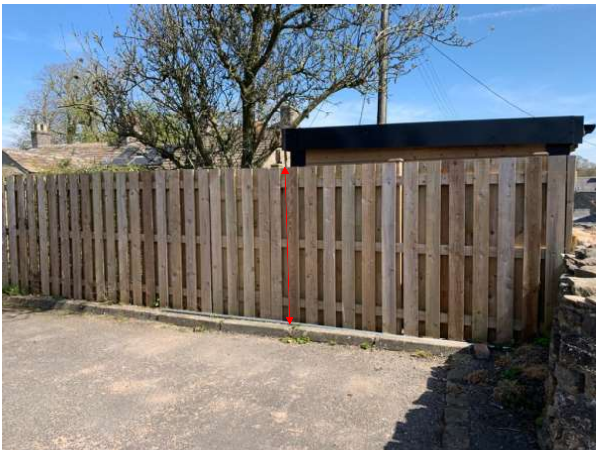
1.85 metre high timber close board fence
