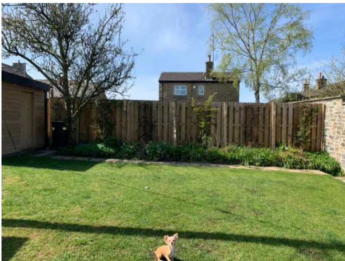
1.85 metre high timber close board fence
