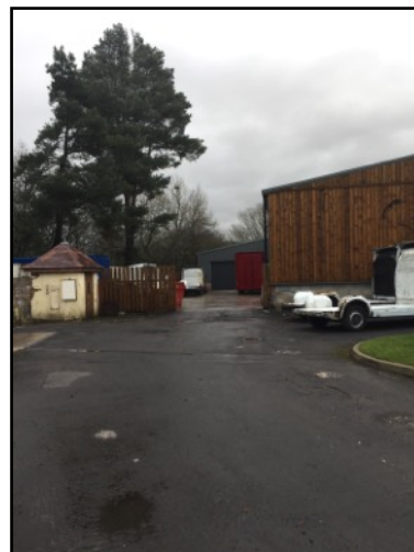
Photograph 4: View looking east towards the service yard area and the front of the new extension
