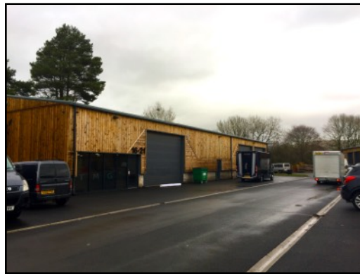
Photograph 2: Front elevation of units 16-21
