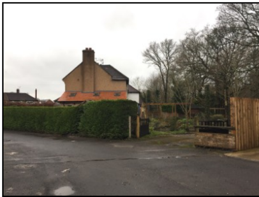
Photograph 1: view looking west to the side elevation of no 1 The Cottages
