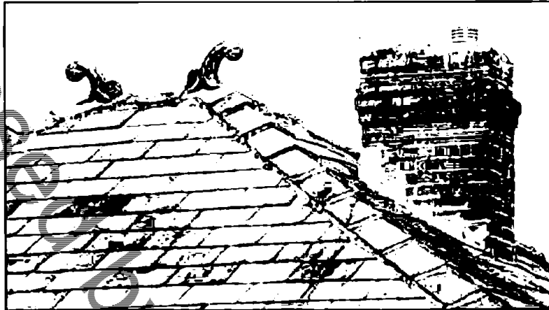
View of roof coverings and lead flashing on chimney, all good condition with few gaps visible.
