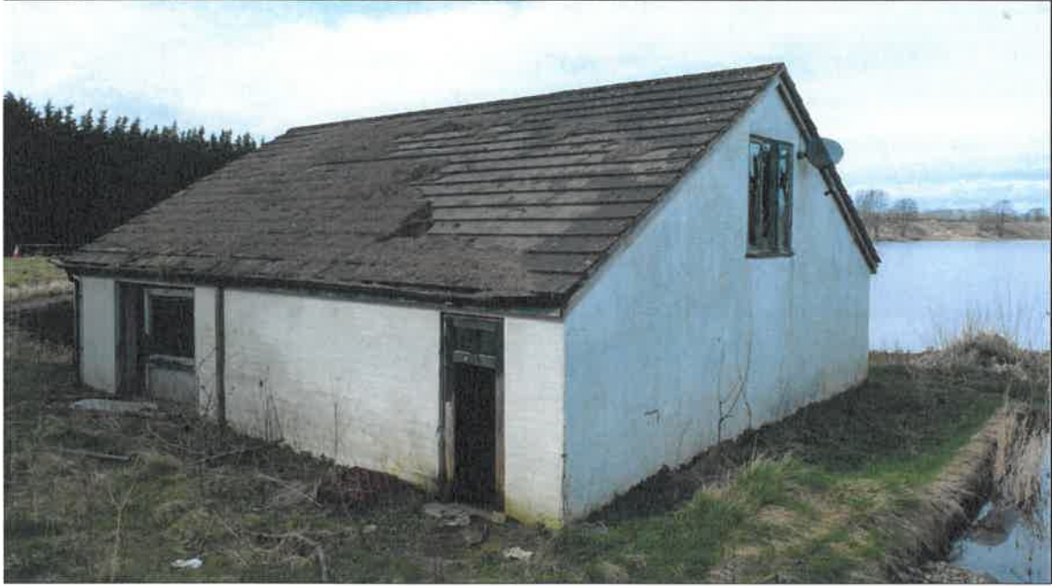
Disused lakeside building, subject to damage from vandals. Frequent signs of nesting birds, including several disused nests. This building has high potential for use by nesting birds. April 2021
