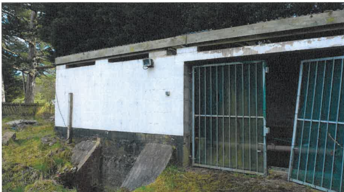
Former hatchery building – previously used for nesting by grey wagtails. This building has high potential for use by nesting birds. April 2021
