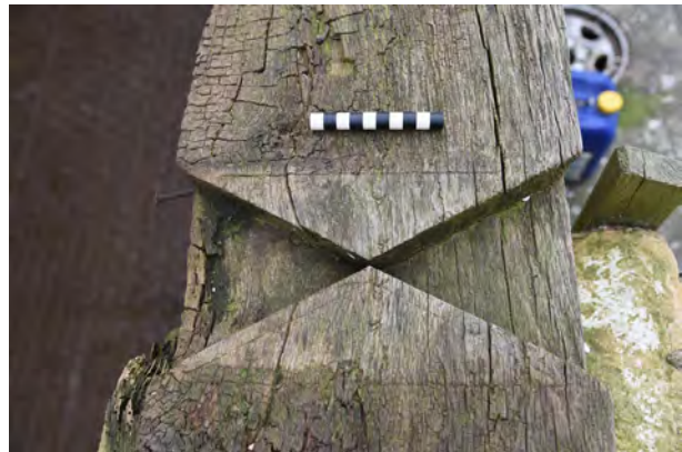
Plate 19 Upper part of wall plate showing notches for tie beam
