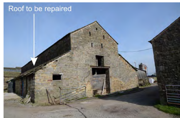
Plate 3 Southeast elevation of the barn
