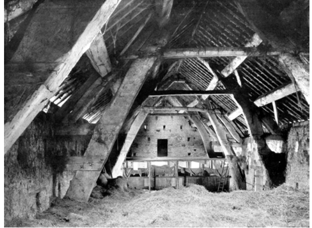
Plate 6 Interior of the 'Shireburn Barn', 1927 (Stonyhurst Magazine)
