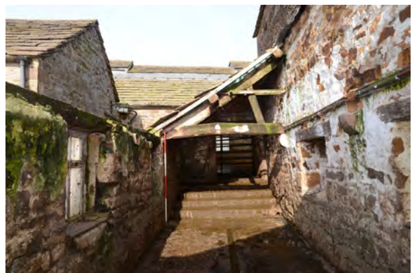
Plate 18 Interior of the north end of the outshut on southwest side
