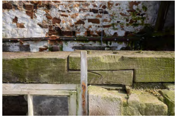
Plate 20 Wall plate towards the north end of the southwest outshut
