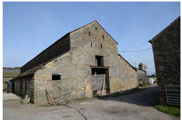
Plate 17 Southeast elevation of the barn
