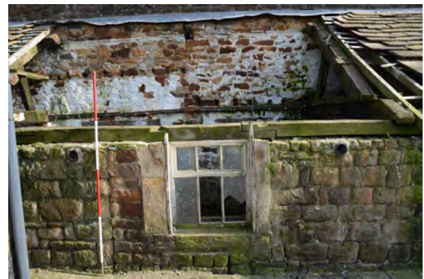
Plate 15 Window inserted in doorway, southwest elevation
