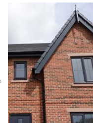
Brick on edge detail
