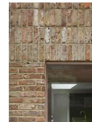
Brick on edge detail
