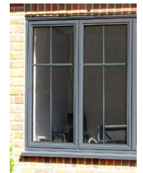
Brick on edge detail
