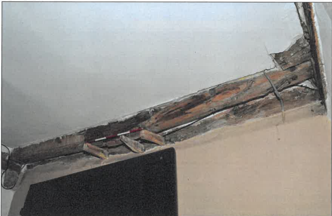
Photo 14: Beam 3, dining room
