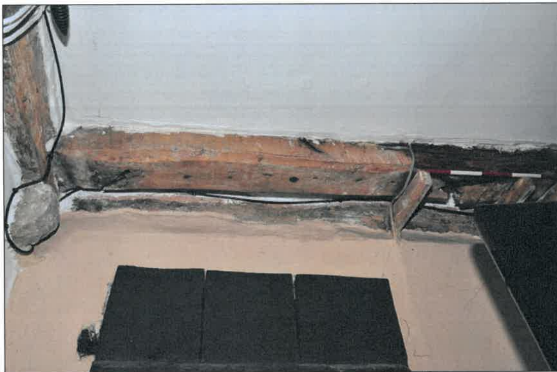
Photo 15: Beam 3, dining room
