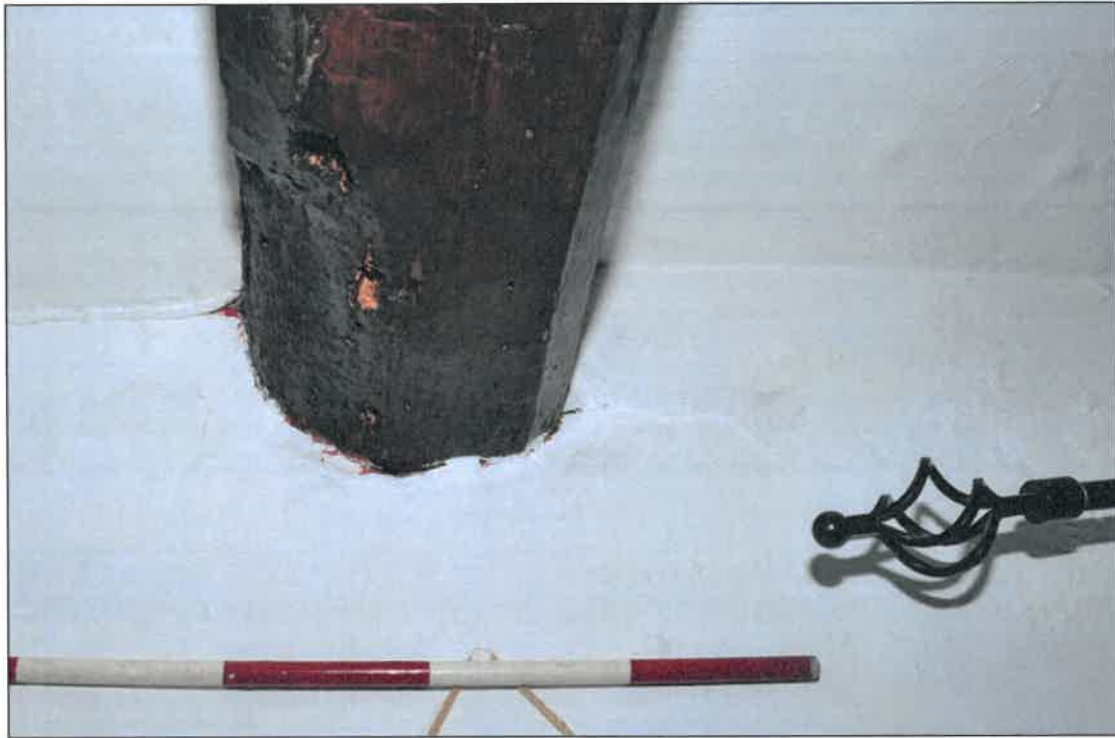
Photo 11: Beam 2, middle of lounge/living room
