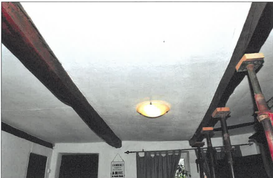
Photo 6: Beams 1 (right) and 2 (left), in lounge/living room
