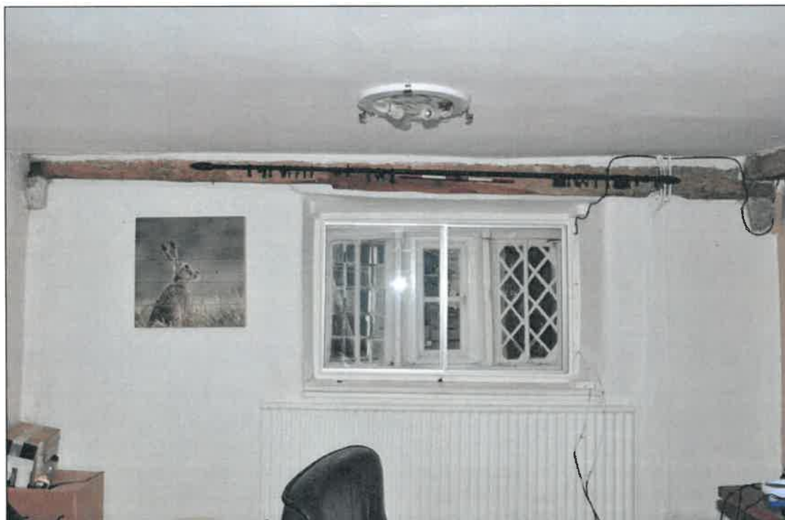
Photo 20: Beam by outer wall of dining room
