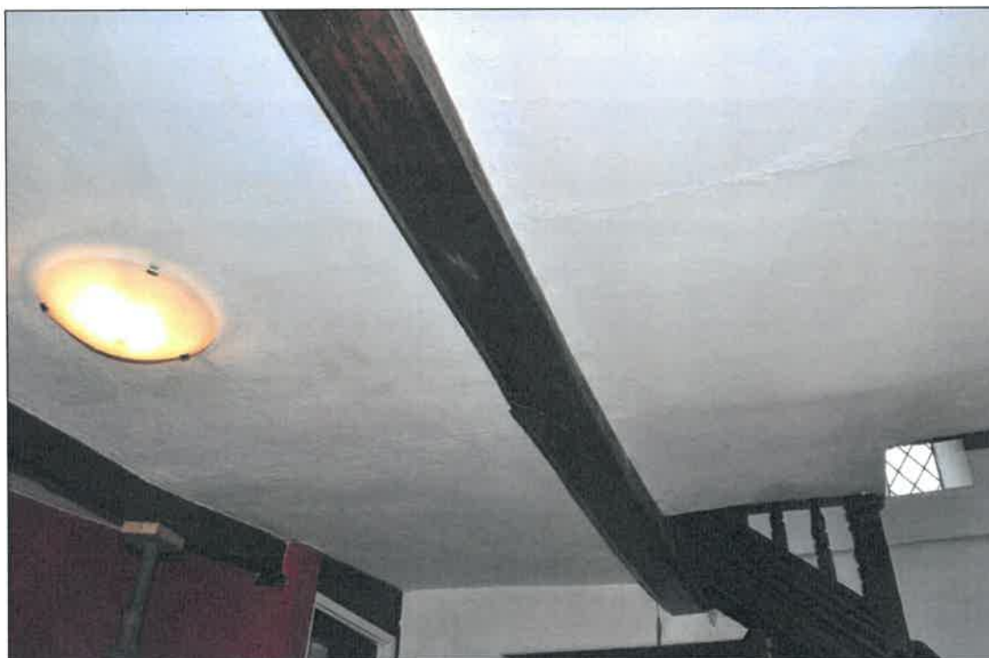
Photo 8: Beam 2, middle of lounge/living room
