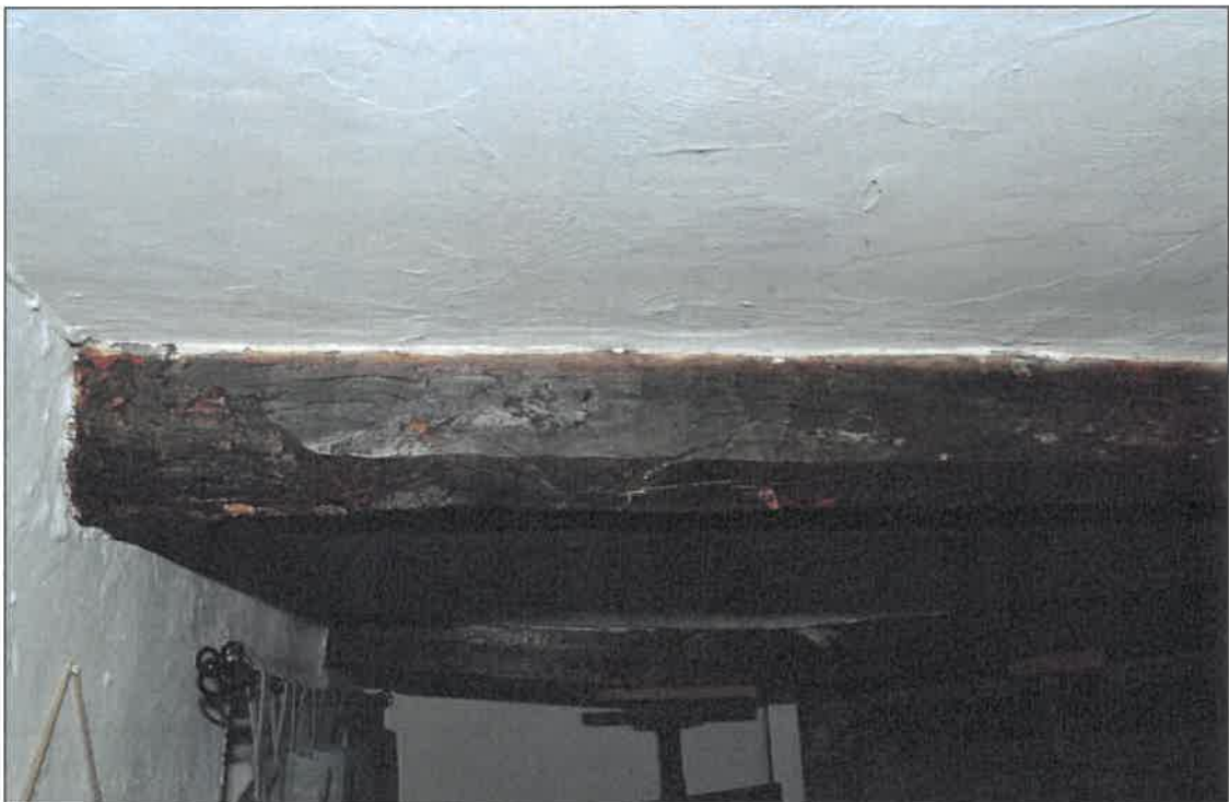
Photo 10: Beam 2, middle of lounge/living room
