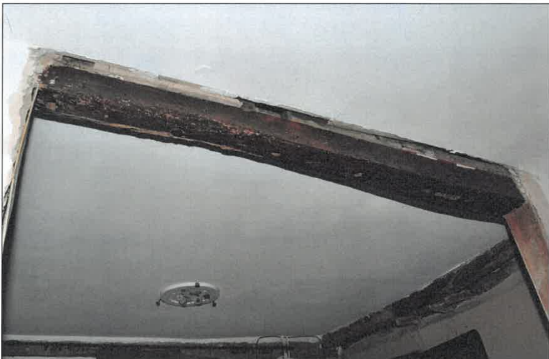
Photo 18: Beam over partition between dining room and study
