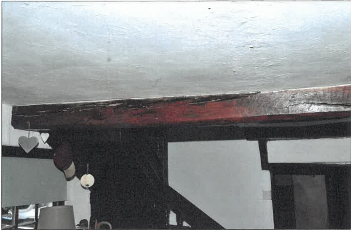
Photo 9: Beam 2, middle of lounge/living room
