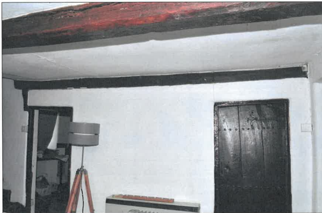
Photo 12: Beam over partition between lounge/living room and study/dining room
