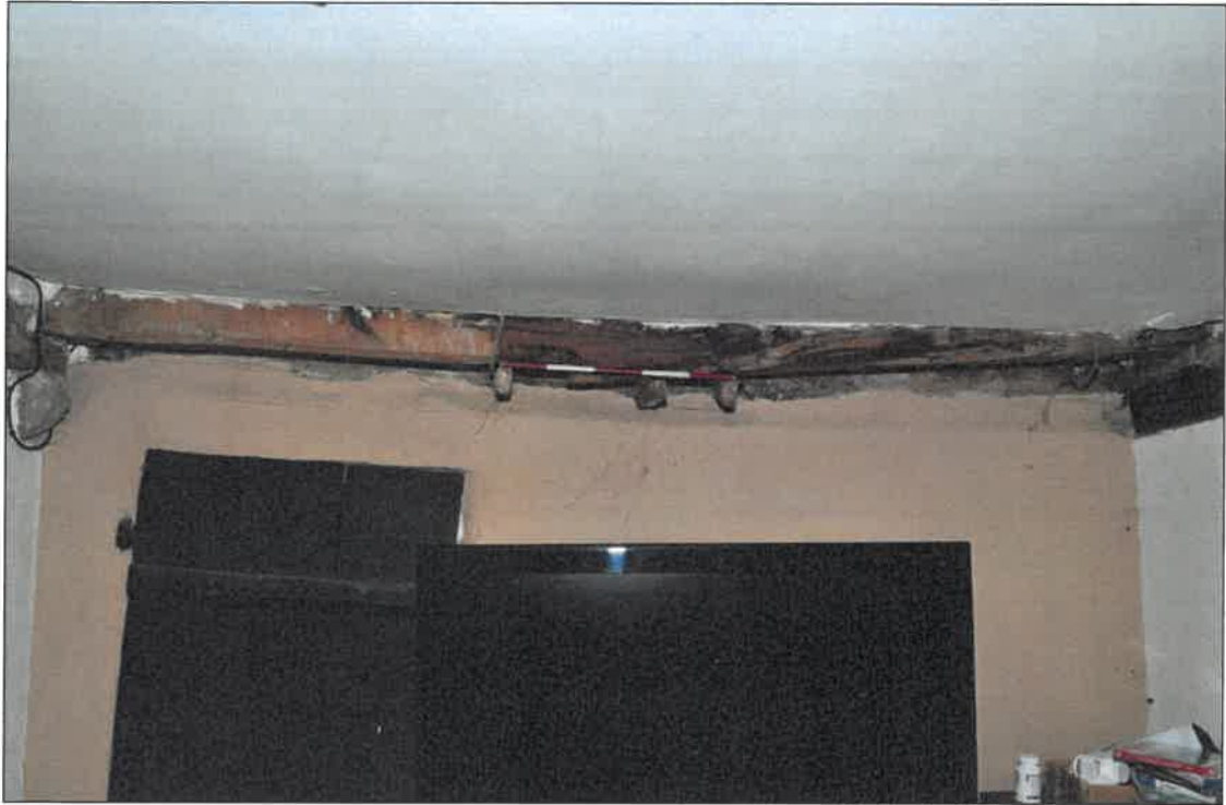
Photo 13: Beam 3, dining room
