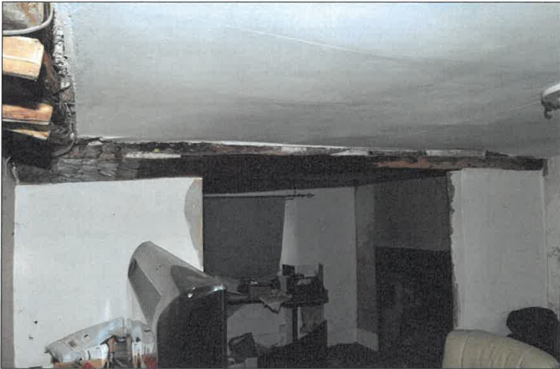
Photo 17: Beam over partition between dining room and study
