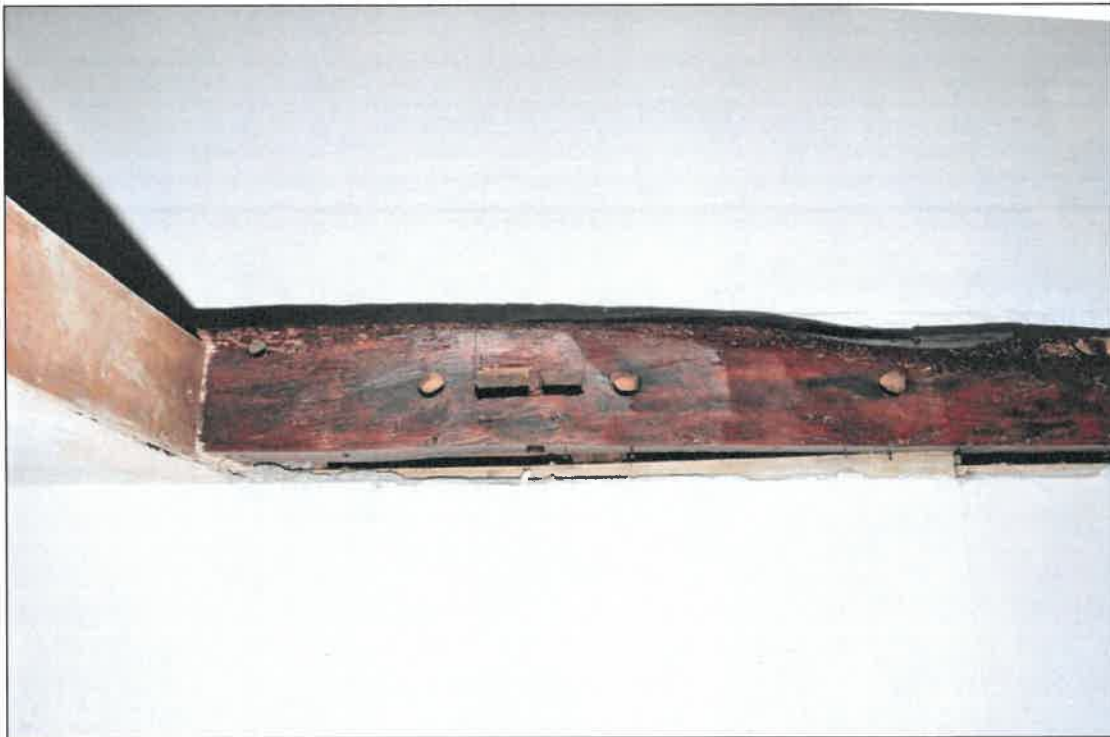
Photo 19: Beam over partition between dining room and study
