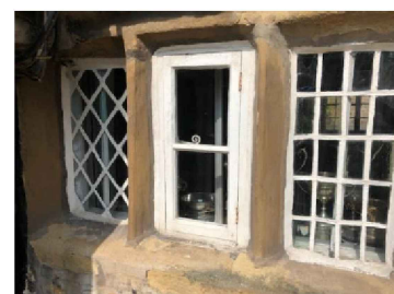
WINDOW 3 Central Casement
