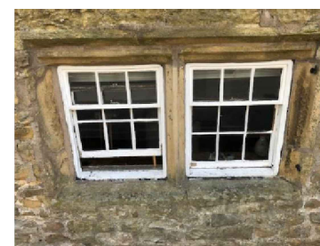
WINDOW 1 Both sash windows
