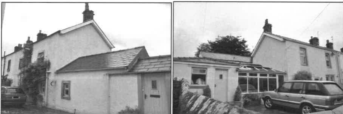
Front (lhs) and rear (rhs) elevations of 90 Regent Street showing two storey building with adjoining single storey extensions
