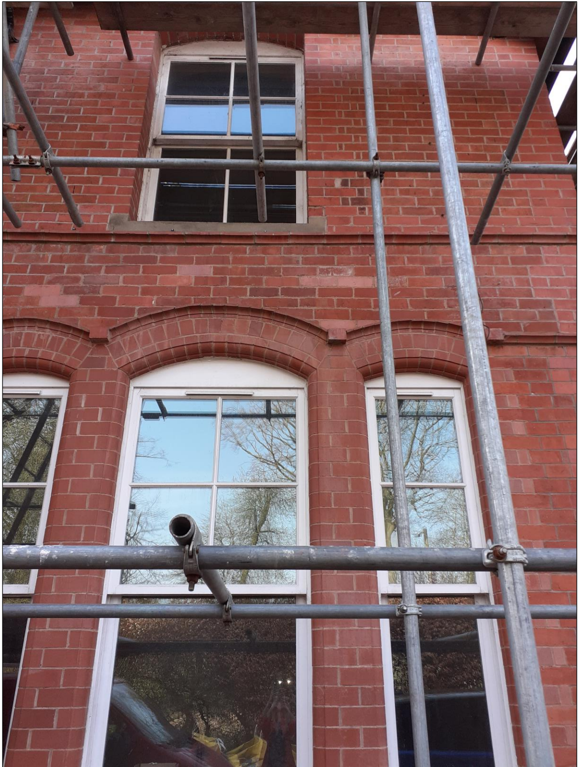
4 Brick detailing around windows and sting courses.
