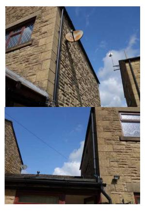
The property consists of a semi-detached stone built two storey house with double pitched tiled roof. External walls are pointed and in good general condition, with well pointed gable ends. Roof tiles are close fitting with ridge tiles pointed and well sealed. Fascia boards are close fitting.
