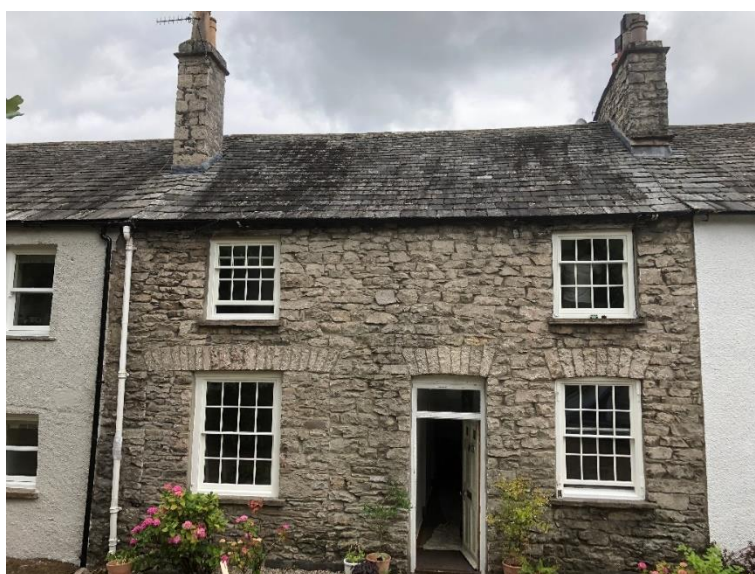
Picture 10 - Example of Cottage Renovation in Kendal using double glazed sliding sash windows by ECOSASH
