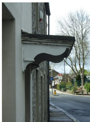
Picture 9 - Timber hood to #13
