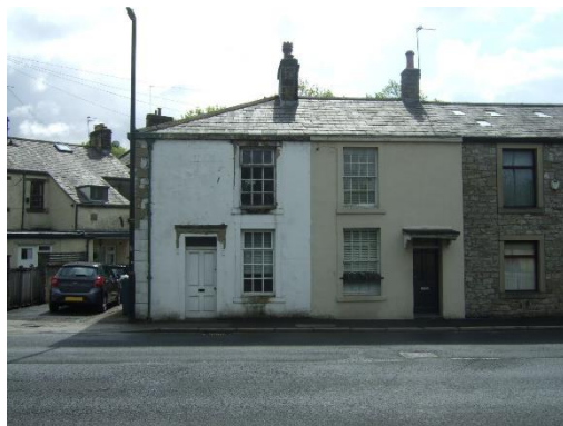
Picture 4 – West elevation along Railway View Road
