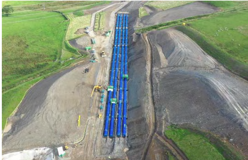
Example of open-cut trenching
