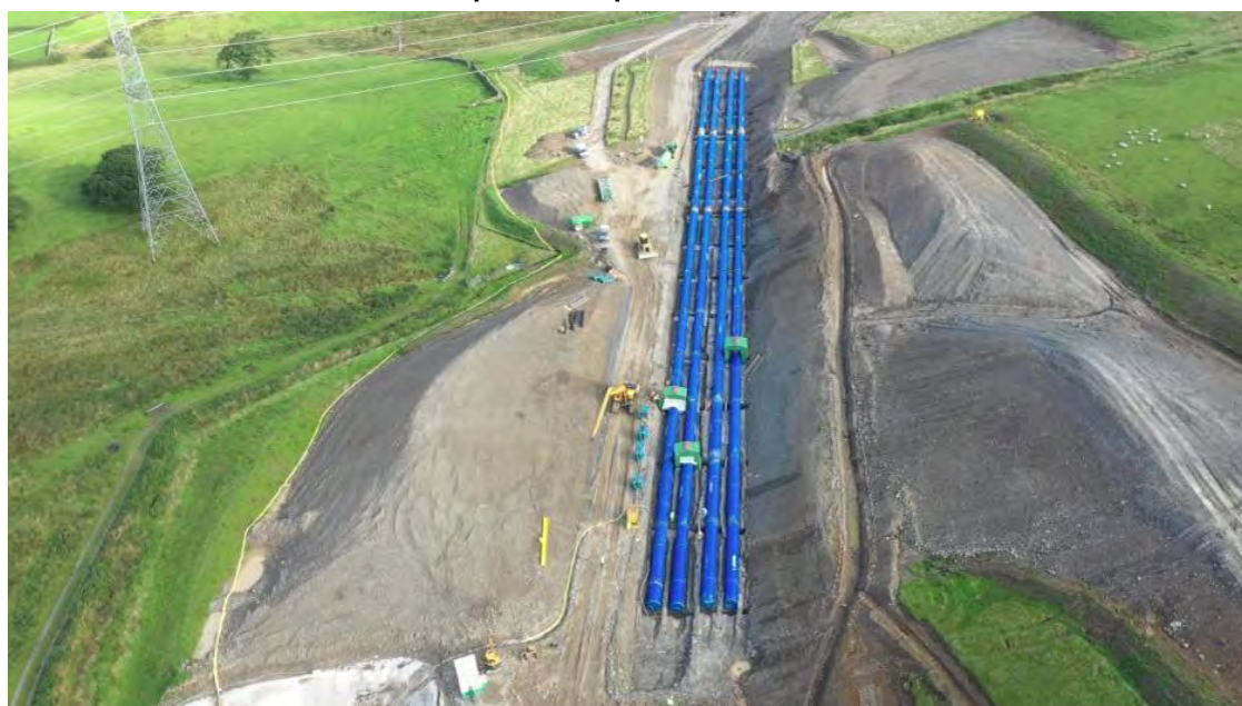
Illustration 3.6: Example of an open-cut construction area
