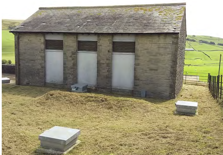
Illustration 3.5: Typical valve house building – rural setting
