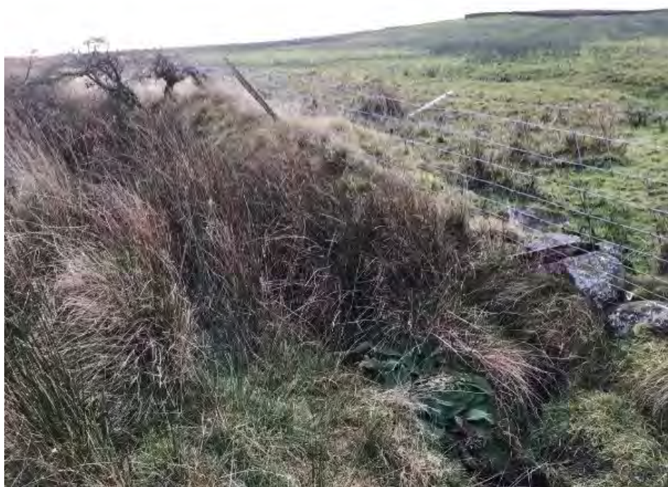
Illustration 2: Upstream view from right bank showing riparian vegetation
