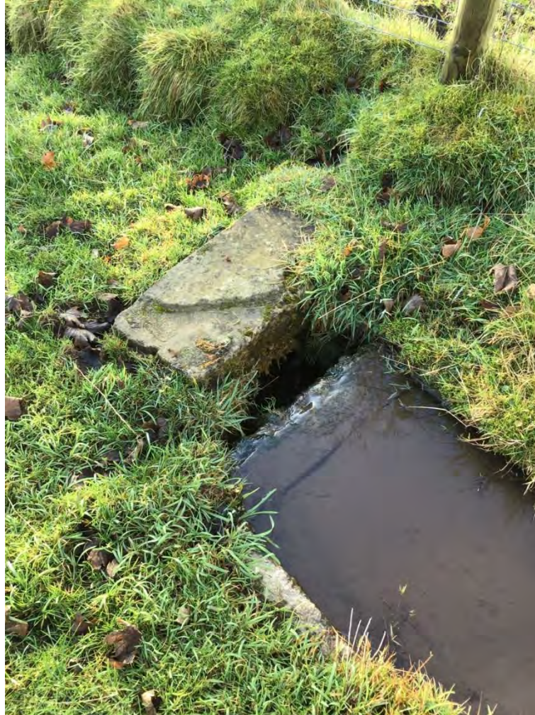
Illustration 4: Downstream view of culvert inlet
