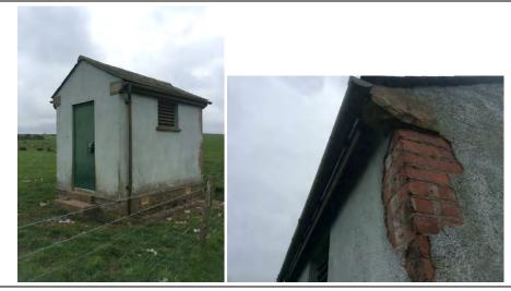
Single storey, small brick operational building with concrete render which is peeling/falling off (no significant crevices). The building has a pitched, slate roof and timber louvred windows on the northern and southern elevations. The roof edge is filled with mortar. Hirundine nests observed on the eastern corner and northern elevation. The building is assessed as having negligible bat roosting potential.
