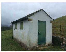
A single-storey rendered United Utilities building with a pitched slate roof. There are gaps present beneath the ridge tiles on the southern elevation and numerous raised roof slates. There are also gaps along the roof verges at both gable ends. There is damaged brickwork on the western gable. Connectivity to wider landscape is limited to scattered scrub on the exposed field boundaries. Overall low bat roosting potential. No evidence of hirundine nests.
