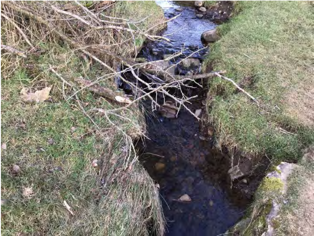
Illustration 4: Upstream view of step and woody debris
