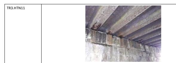
Railway underpass bridge. Comprising steel girders and stone abutments. The stone abutments are well-sealed; however, gaps extend between the steel girders at the top of the stone abutments towards the back wall. These are suitable for use by roosting bats. Further survey may be required if impacts to the bridge are anticipated. The gaps are also suitable for use by nesting birds. The bridge is single span and narrow, with bare ground / species-poor semiimproved grassland beneath.
