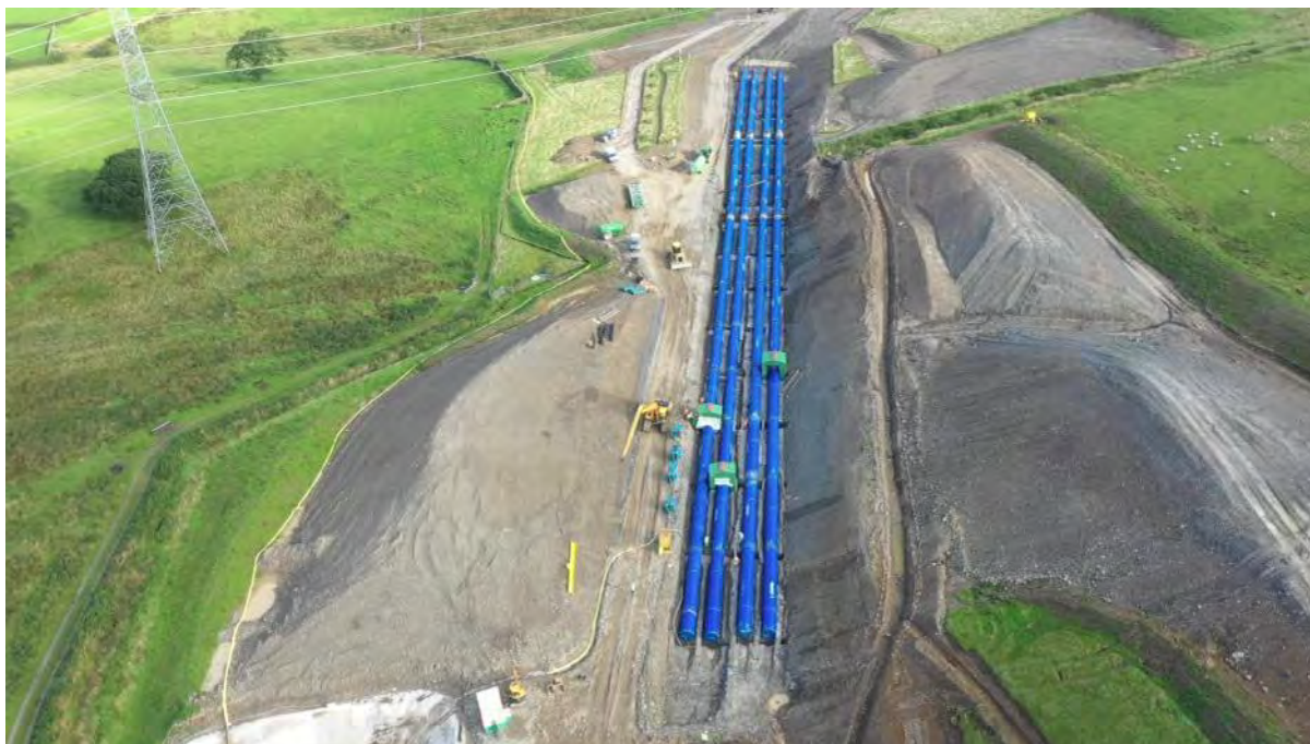
Illustration 3.6: Example of an open-cut construction area
