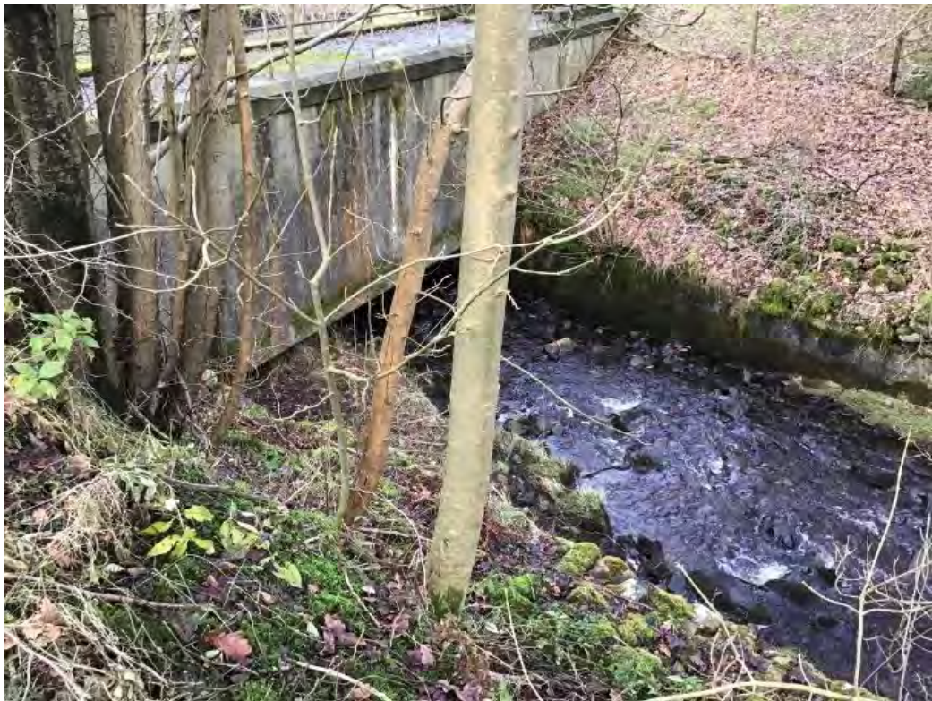
Illustration 3: Downstream view. Haweswater aqueduct pipe bridge
