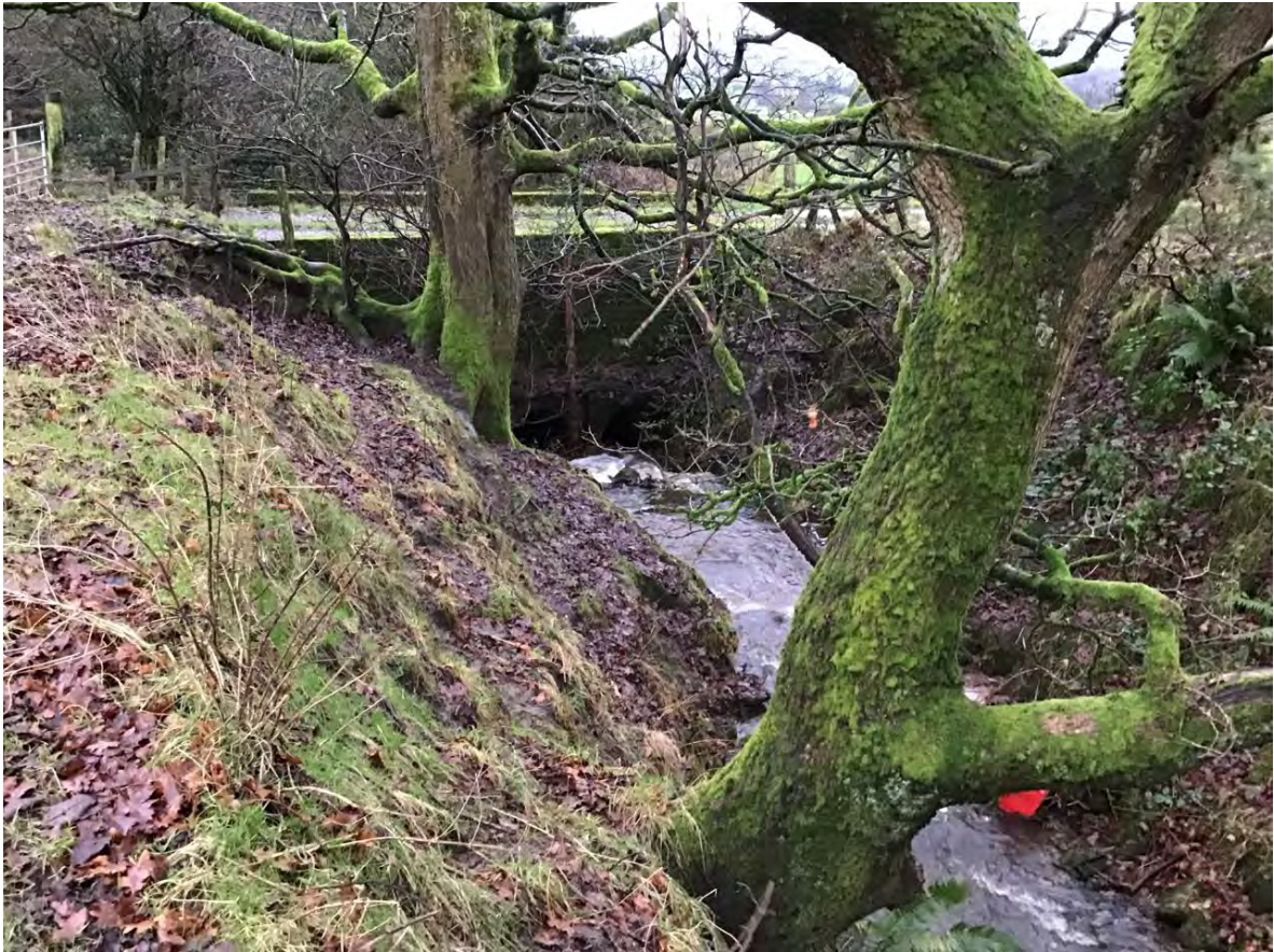
Illustration 11: Upstream view of culvert
