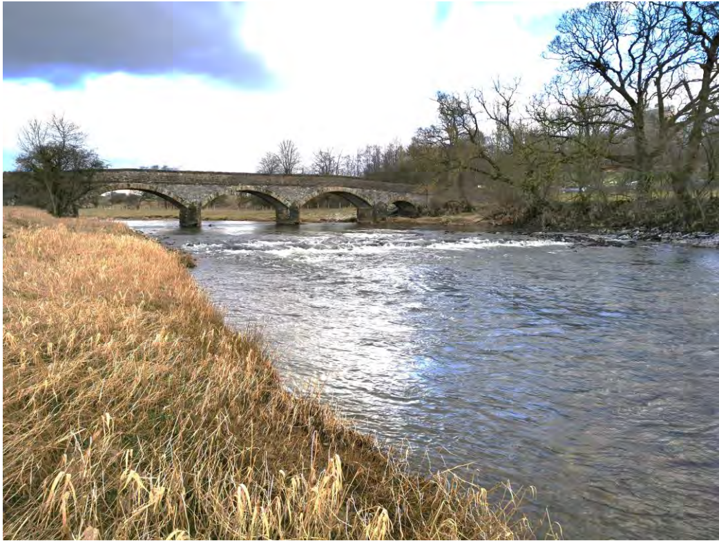
Illustration 1: Upstream view of road crossing and step
