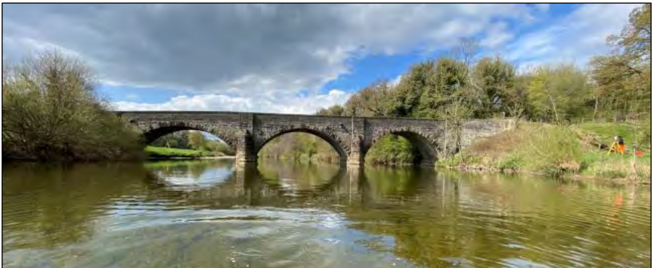
Figure 4-4: Site photograph of Waddington Road bridge (facing downstream).
