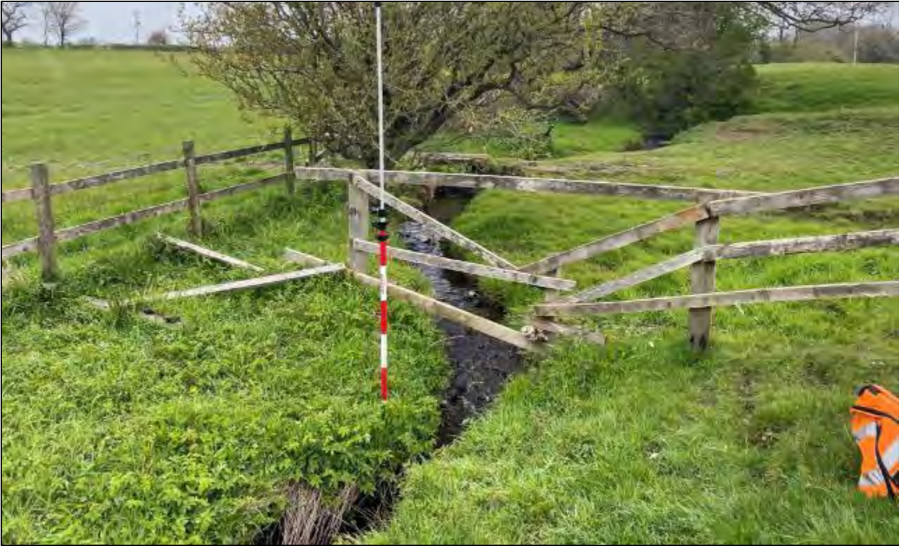
Figure 4-10: Site visit photograph facing downstream, cross-section GRE_1765.
