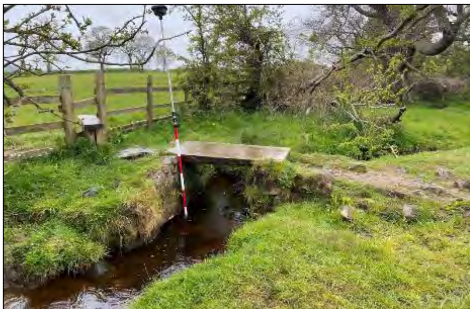
Figure 4-12: Site photograph of Farm Bridge (facing downstream).
