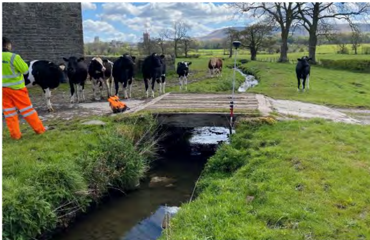
Figure 4-16: Site photograph of Farm Bridge (facing downstream).
