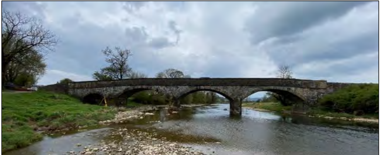
Figure 4-3: Site photograph of West Bradford Road bridge (facing downstream).
