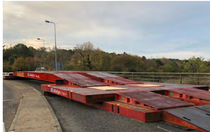
EXAMPLE OF OVERBRIDGING TEMPORARY WORKS
