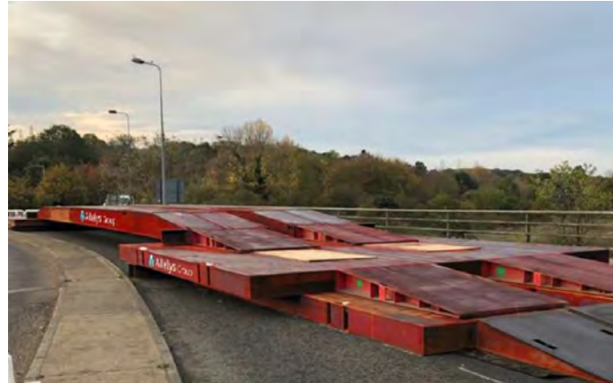
EXAMPLE OF OVERBRIDGING TEMPORARY WORKS
