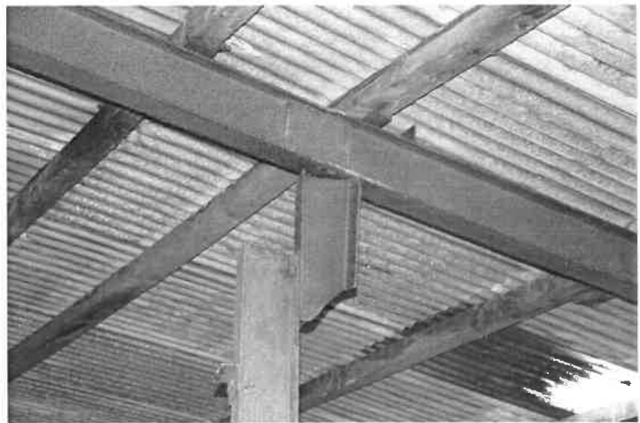
Plate 22 Showing a typical intermediate, internal, Column-Beam Connection of the Pen
