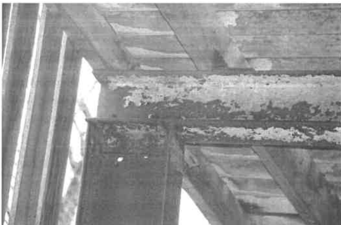
Plate 11 Showing the Front Eaves Portal Frame Connection
