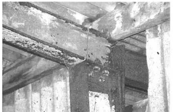
Plate 12 Showing the Rear Eaves Portal Frame Connection
