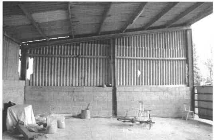
Plate 10 Showing the Internal South-East Elevation
