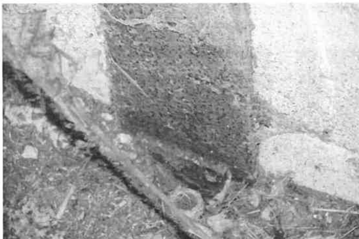
Plate 23 Showing a typical Column Base in the Pen Area
