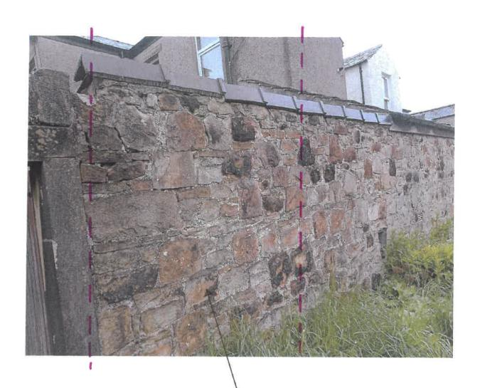
THIS SECTION OF WALL TO BE REMOVED AND REPLACED WITH TIMBER SHED.
