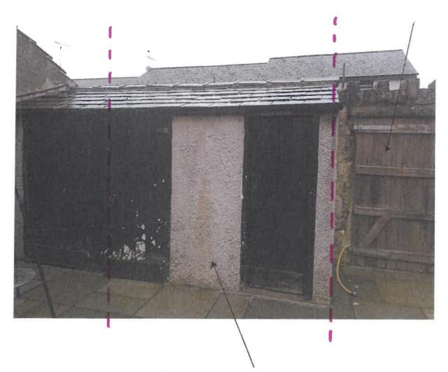
THIS SECTION OF OUTBUILDING TO BE DISMANTLED AND REPLACED BY THE PROPOSED SHED.
