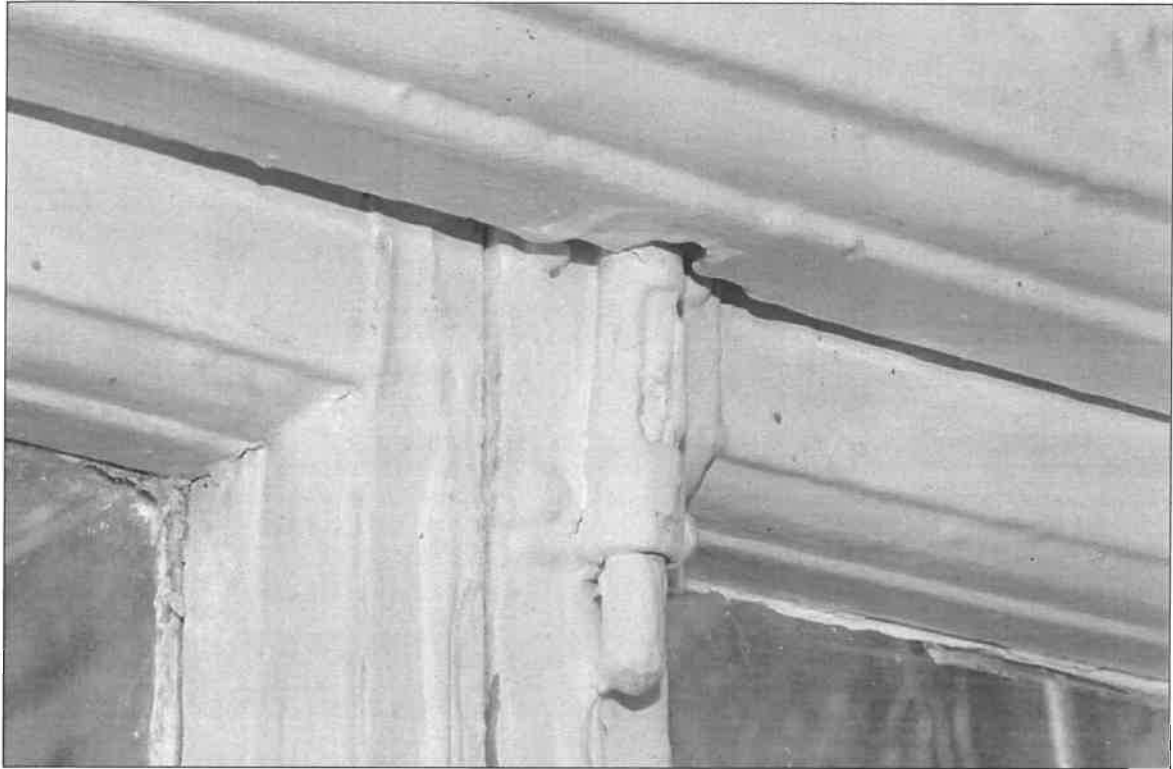
Photo 29: W4, detail of upper bolt
