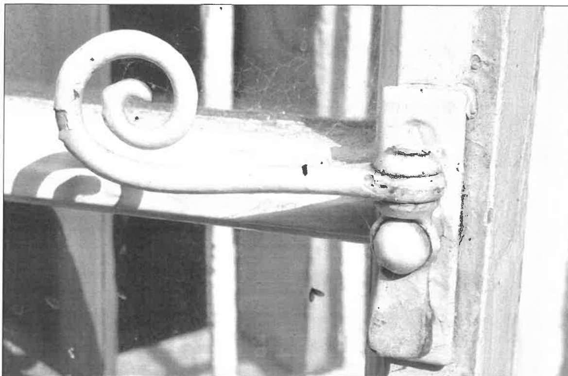
Photo 21: W3, detail of latch
