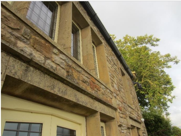
Photo 11: Elevation wall to be covered by Extension 2
