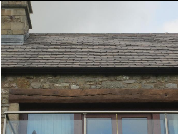
Photo 7: Roof slates above balcony at Extension 1
