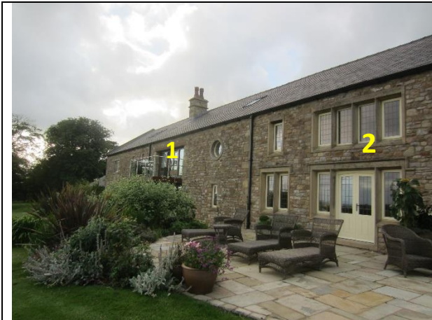
Photo 1: Southern elevation of property showing proposed locations of Extension 1 and 2 and the herbaceous borders
