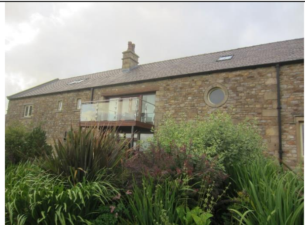
Photo 2: Southern elevation of property showing balcony in position of Extension 1
