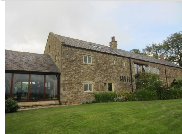
Photo 3: Southern elevation of property showing balcony in position of Extension 1
