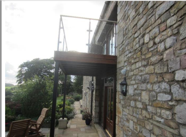
Photo 5: Balcony at Extension 1
