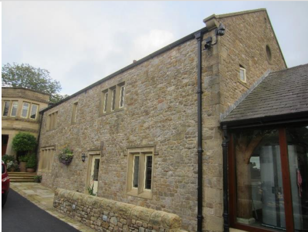
Photo 9: Northern / opposite side of property to Extension 1
