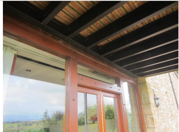
Photo 6: Underside of balcony at Extension 1
