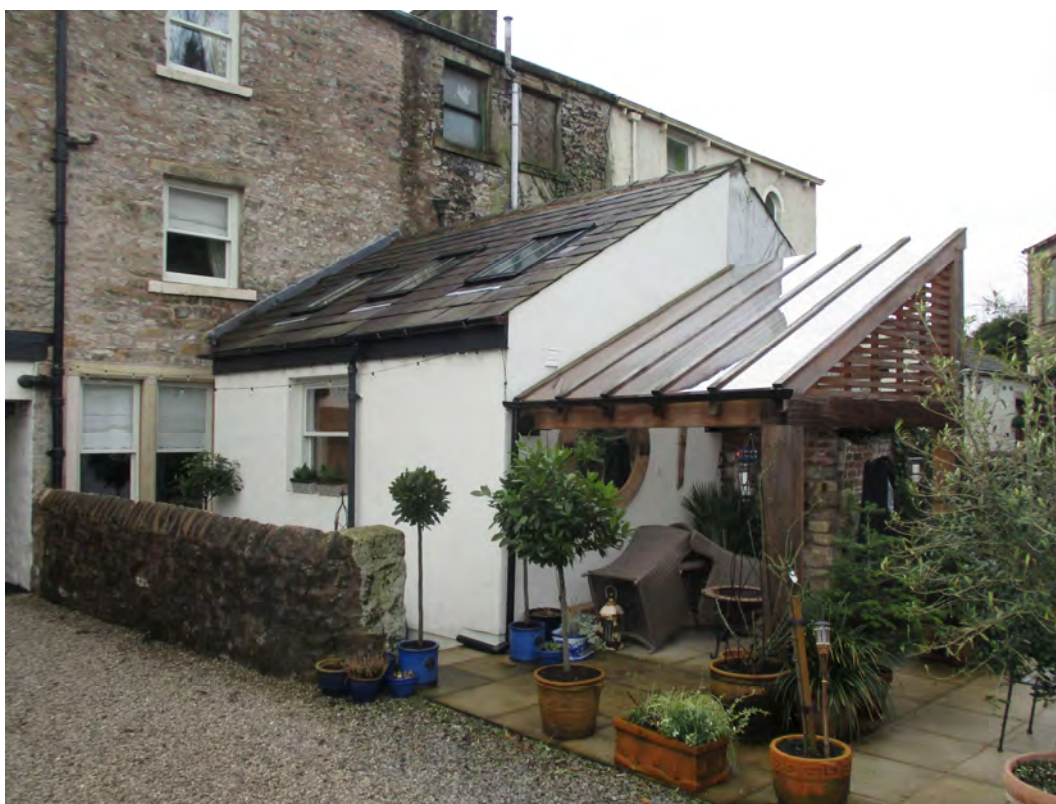
Proposed conservation roof windows to same size and spacing as exists to adjoining half of outrigger
