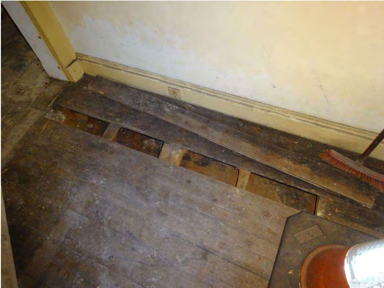
Front Room – Rotten floor joists
