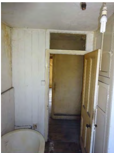
Timber clad partition wall proposed to be removed between bathroom and corridor
