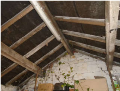
Roof over store room adjacent to wc's.
