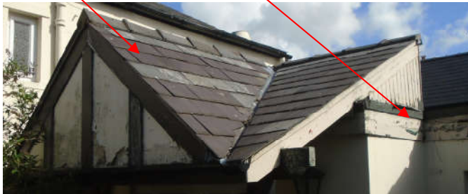
False roof constructed over flat roof to form entrance canopy
