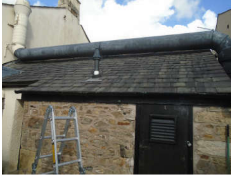
South elevation of the side outrigger.
