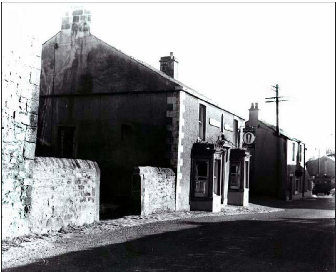
PL10: Photograph of the Buck Inn dating from the mid to late 1950's. Note the visible half-landing window to the east gable end which is now an internal doorway.
