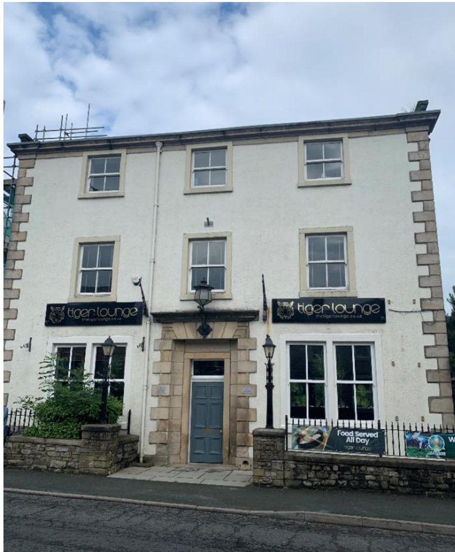
Figure 3. The former Commercial Hotel
