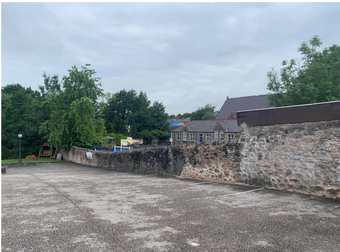
Figure 10. View of School from the former Commercial Hotel Car Park
