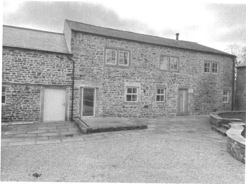
1 Brockthorn north elevation
