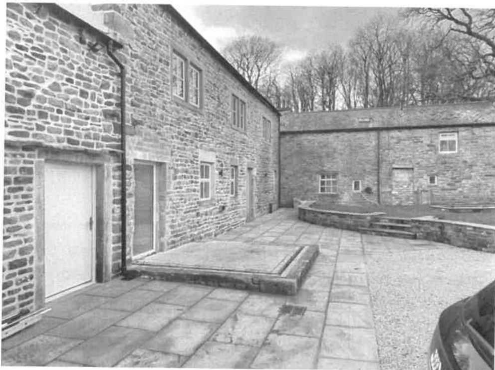
2 Brockthorn north elevation looking west
