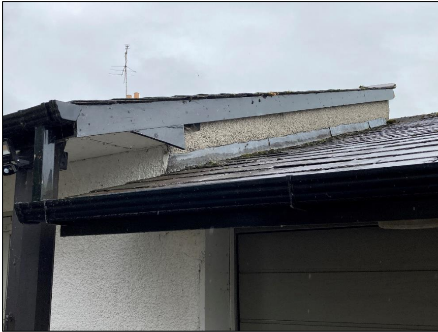
Photograph 6 showing the roof edges and flashing
