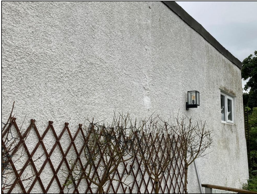
Photograph 2 showing the rear exterior of the garage/store
