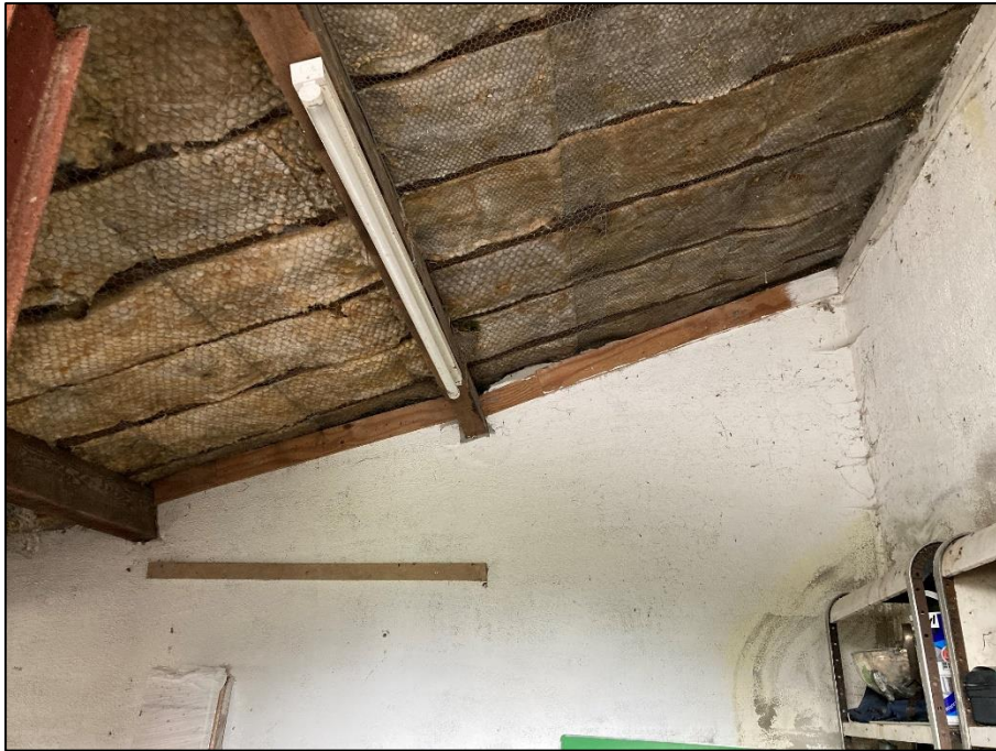
Photograph 9 showing the interior roof of the store
