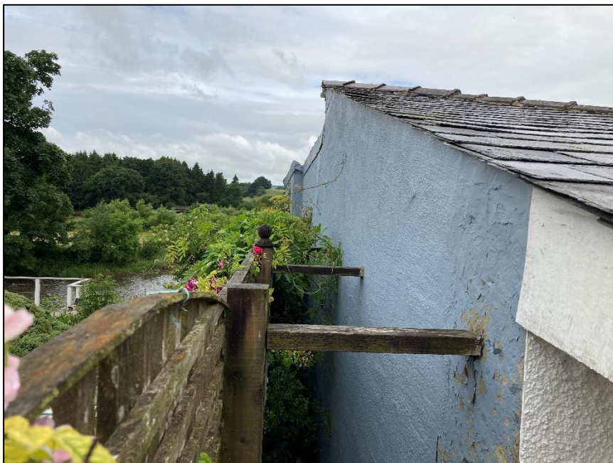
Photograph 5 showing the roof and west-facing edge
