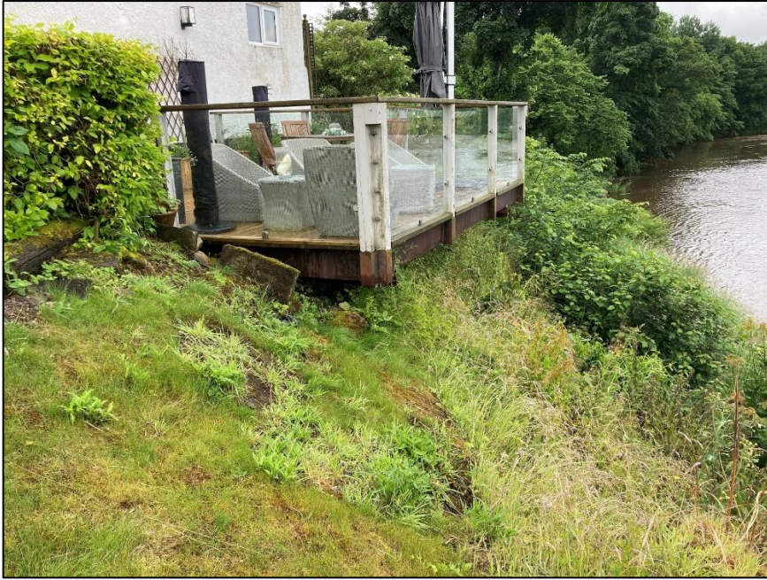
Photograph 12 showing the decking and riverbank
