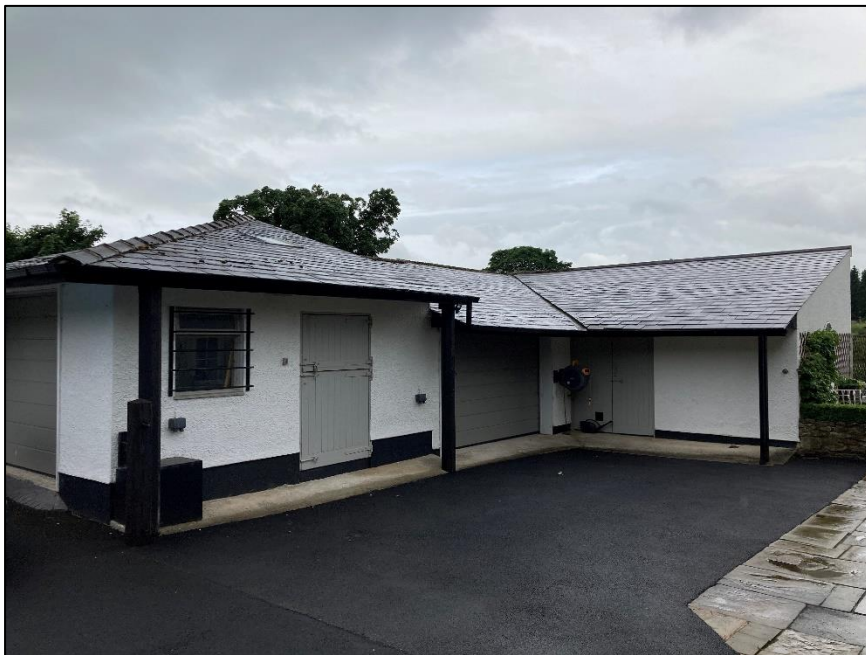
Photograph 1 showing the front exterior of the garage/store
