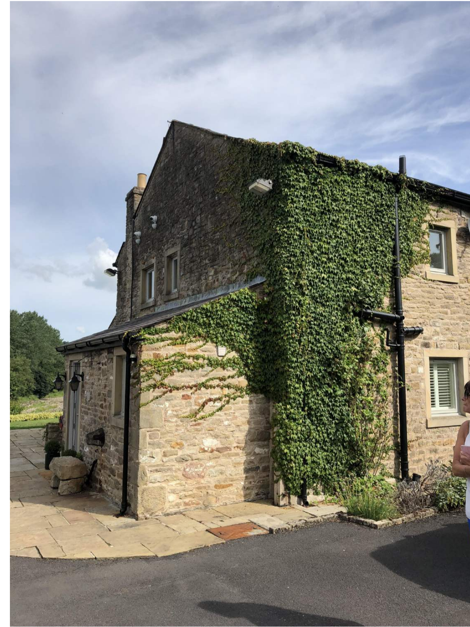
view of the existing house lean-to porch
