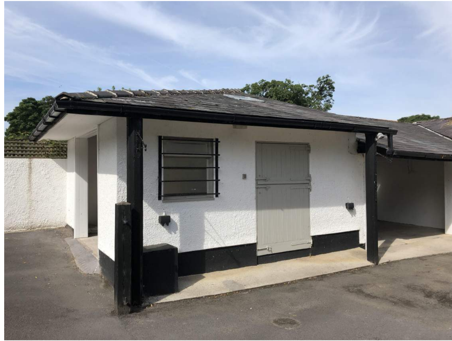
side view of the garage/ store
