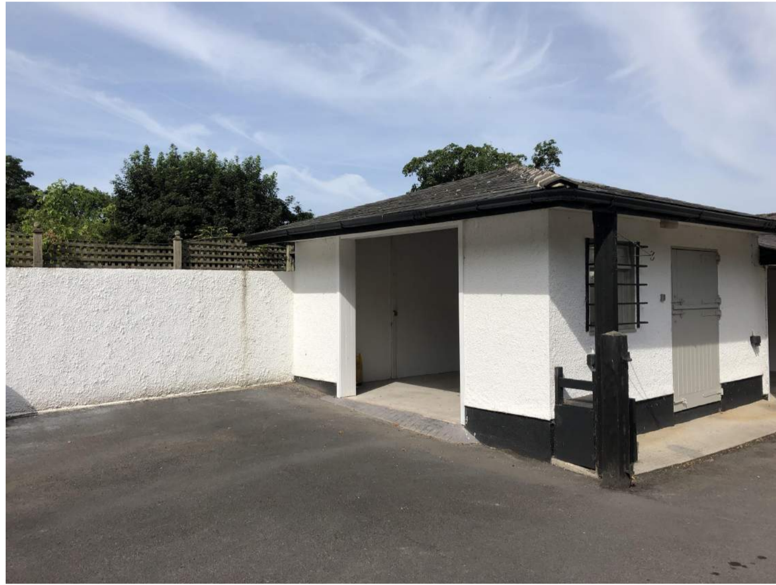
front view of the garage
