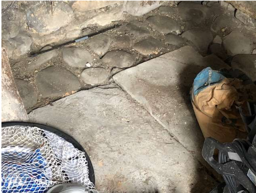
Larger store room with York stone slabs and cobble floor finish
