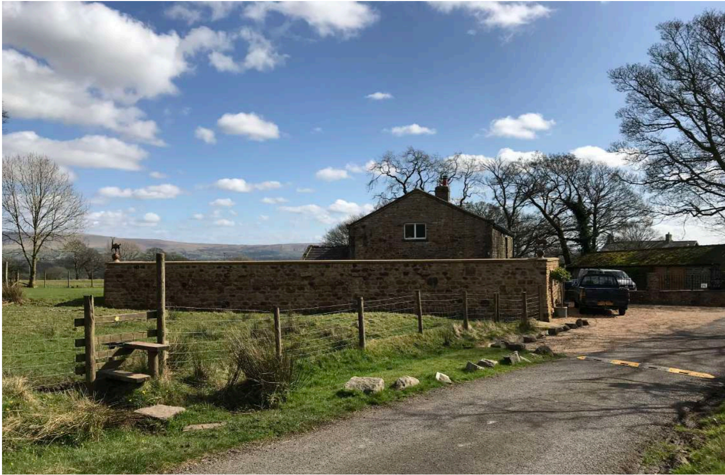
PL02: Photograph of existing barn taken on approach down the private track off Cross Lane.
