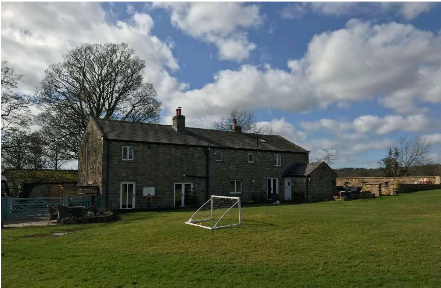
PL04: Photograph of the east (rear) elevation of the existing barn.
