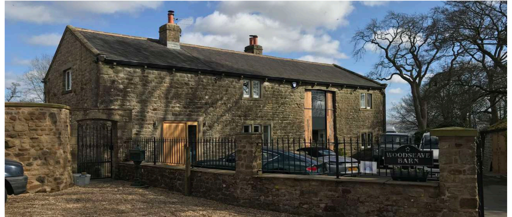
PL06. Photograph of the west (front) elevation of the existing barn taken from the private track off Cross Lane.
