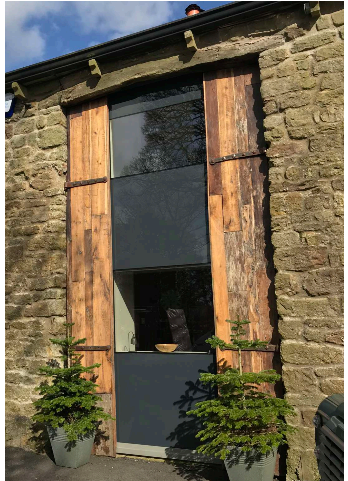
PL08: Photograph of the existing contemporary glazing to the cart opening to the west (front) elevation of the existing barn.
