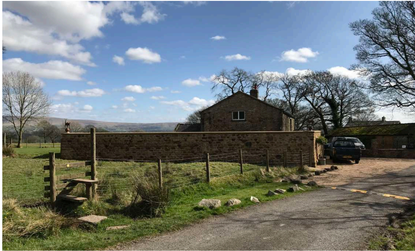
Existing View on approach down the private track off Cross Lane.
