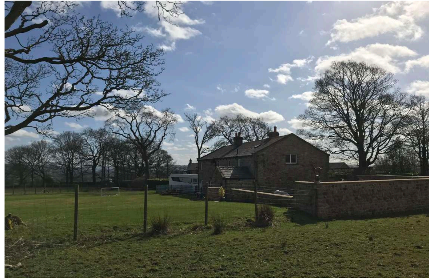
PL03: Photograph of existing barn taken from the public footpath to the north of the site.
