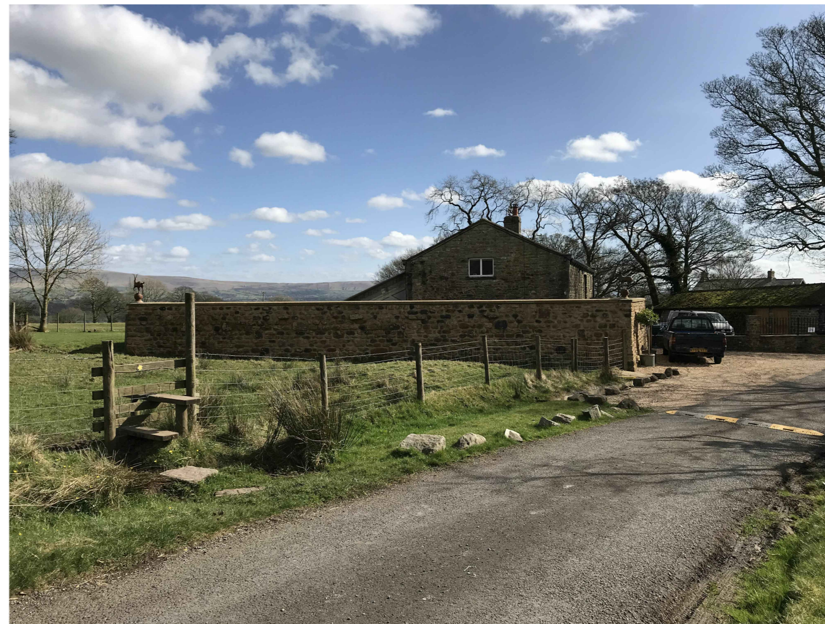
Proposed (Visual 1) on approach down the private track off Cross Lane.
