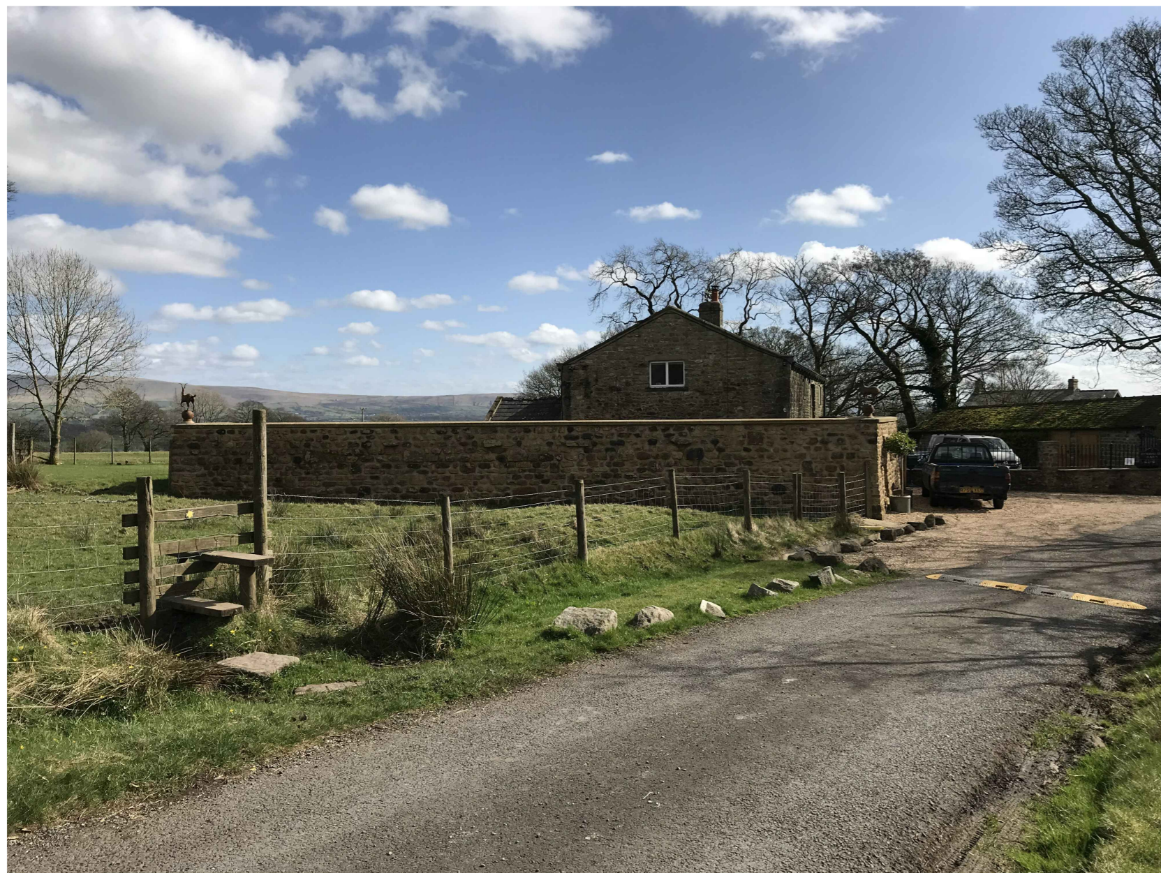
Existing - Photograph of existing barn taken on approach down the private track off Cross Lane.
