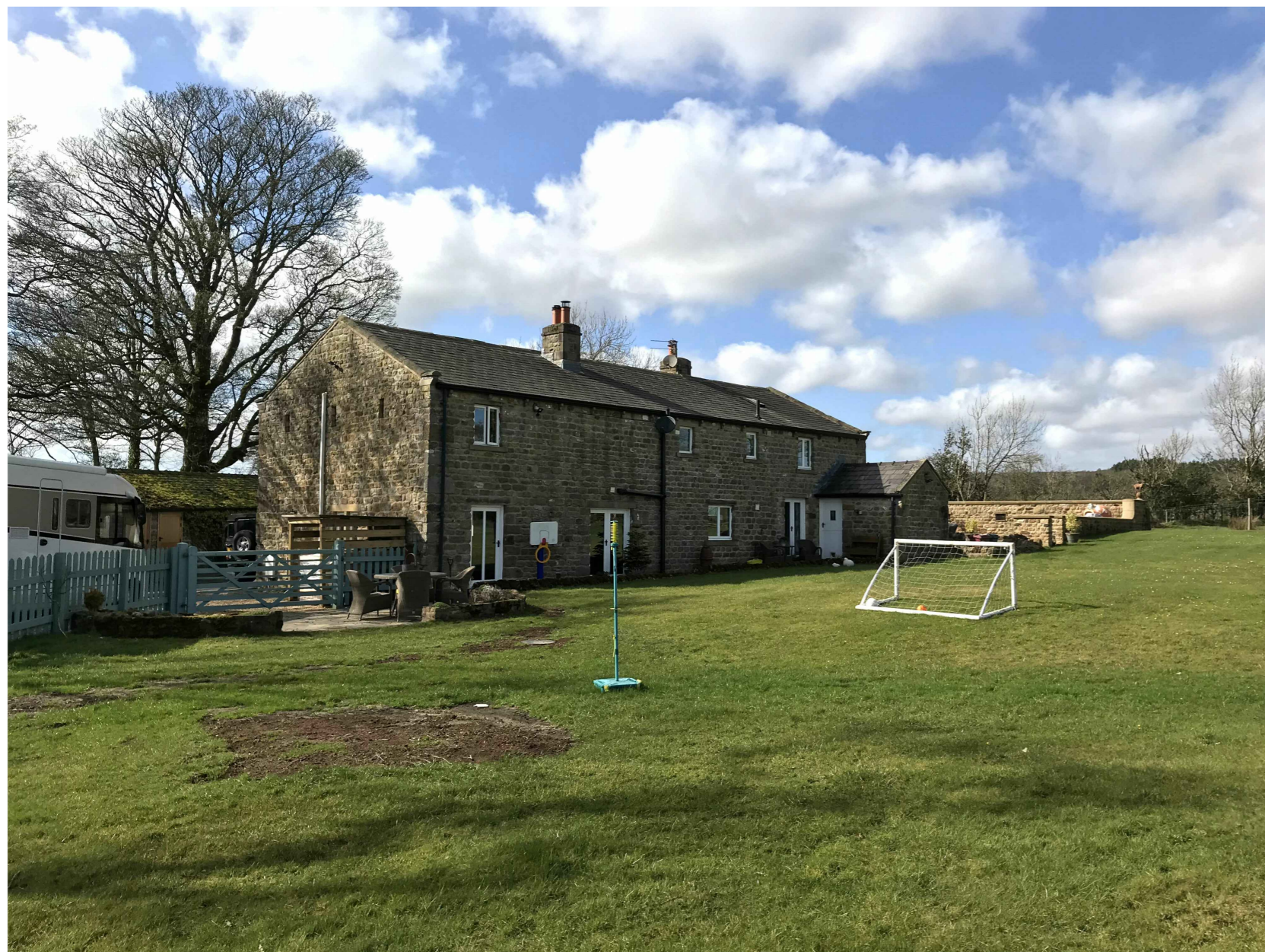
Existing - Photograph of the east (rear) elevation of the barn.
