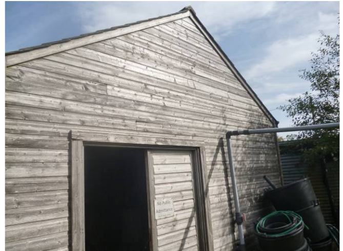
Wooden shed in NE corner with no bat roost potential.
