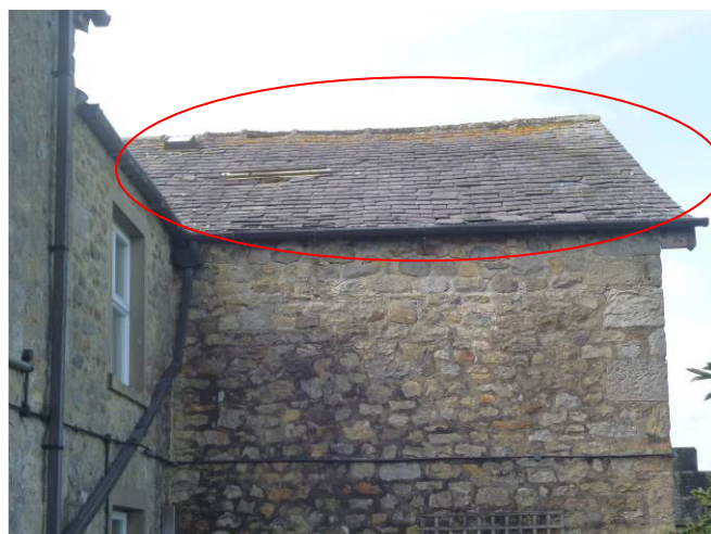
Target Note 7: Northern elevation of barn with multiple potential bat roost features.
