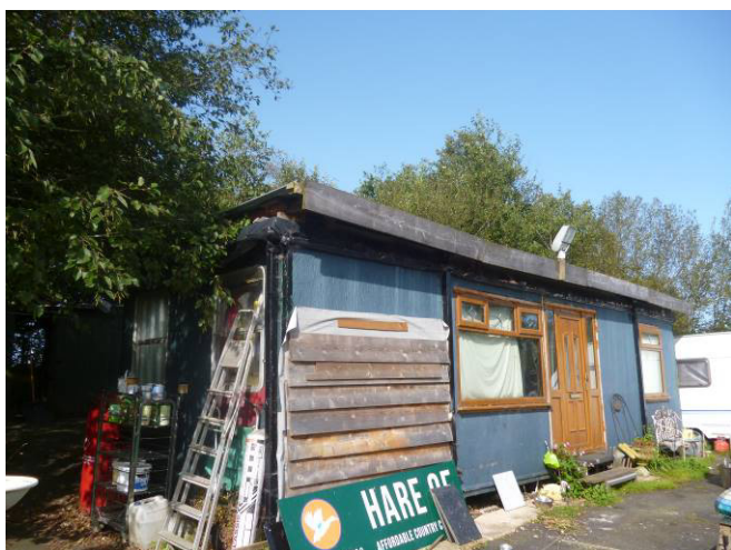
Wooden cabin in central part of site, no bat roost potential.
