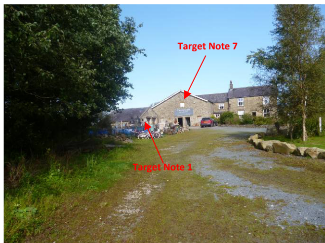
Target Notes 1 & 7: Outbuilding and house / barns with moderate bat roost potential.
