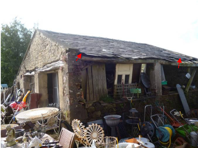
Target Note 1: Outbuilding with multiple potential bat roost features, internal roof with no lining.
