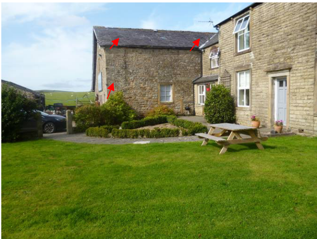
Target Note 7: Barn adjacent to house with multiple potential bat roost features.
