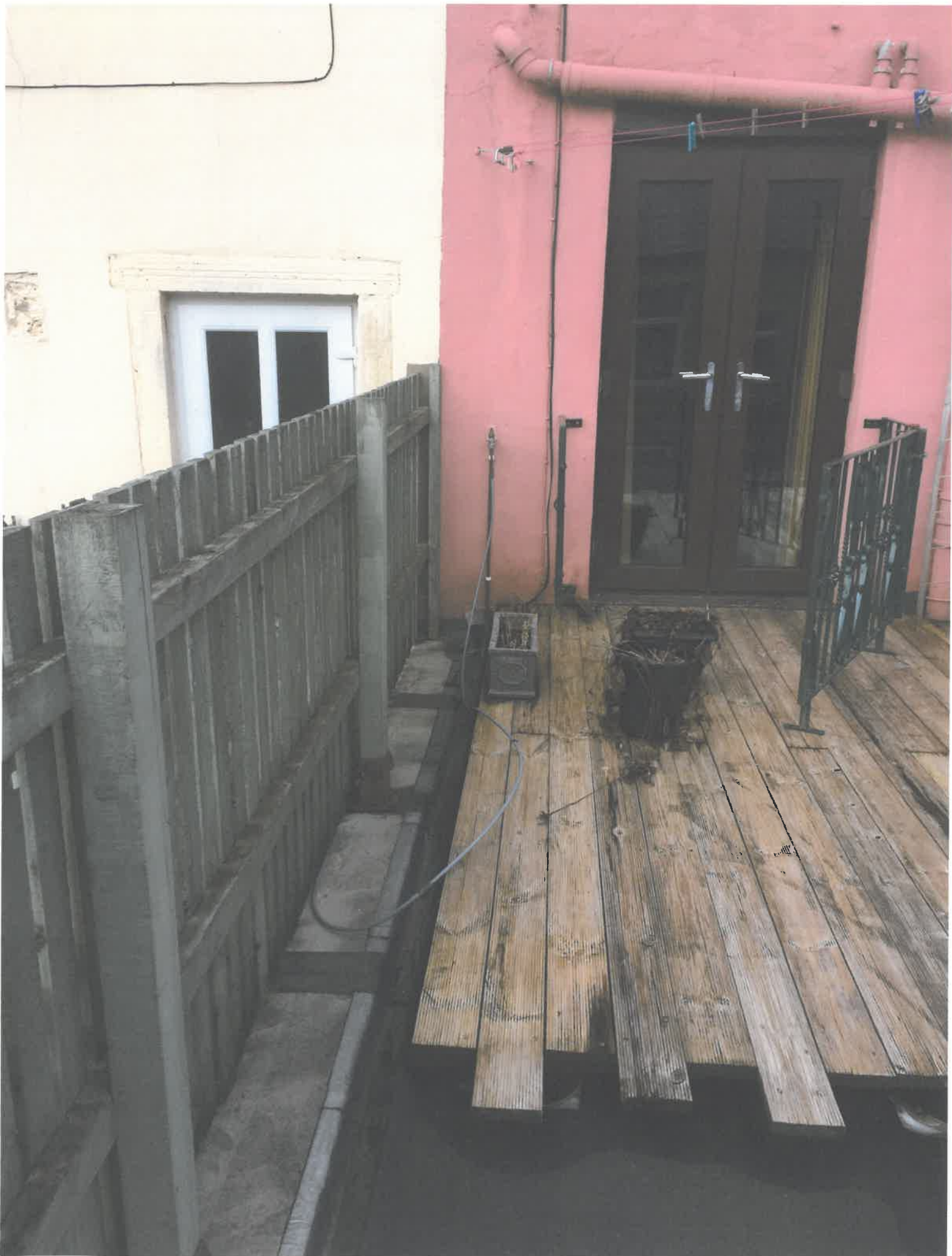
✓ VIEW OF EXISTING FENCE FROM STREET 48" HIGH.
