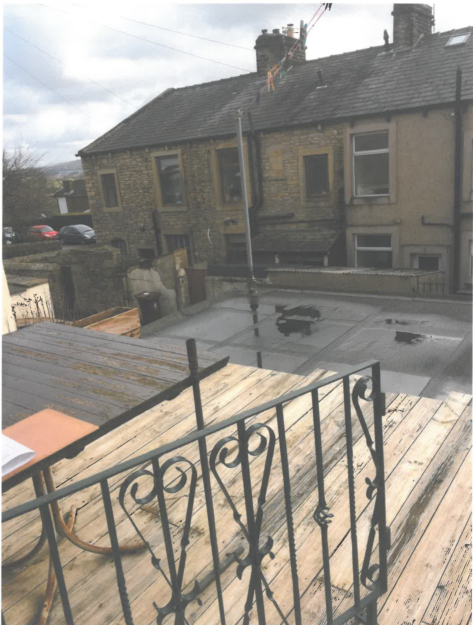
3/1 VIEW GARAGE ROOF FROM No 5 WINDOW.
