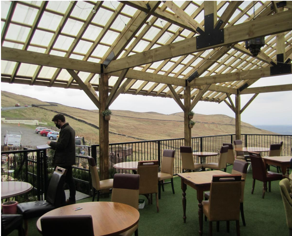
Image 1 Proposed timber canopy with exposed beams provides shelter and retains views across the landscape.
