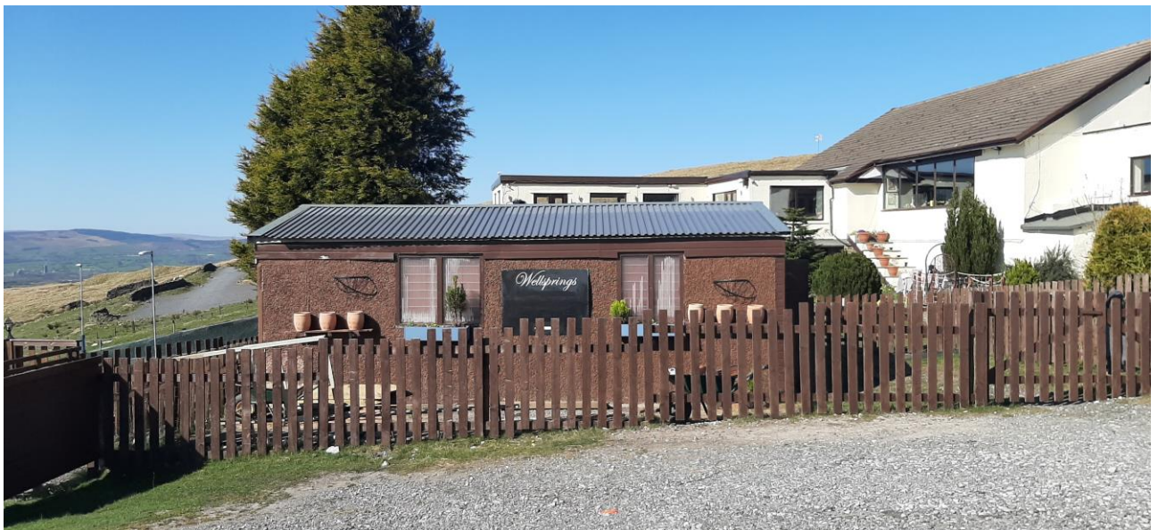
Image 5 View from the car park prior to the canopy being installed.
