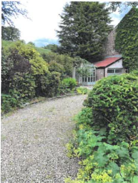
Photo 1: view of the shed from driveway
