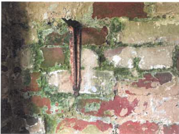
Photo 3: view of the inside wall of the shed
