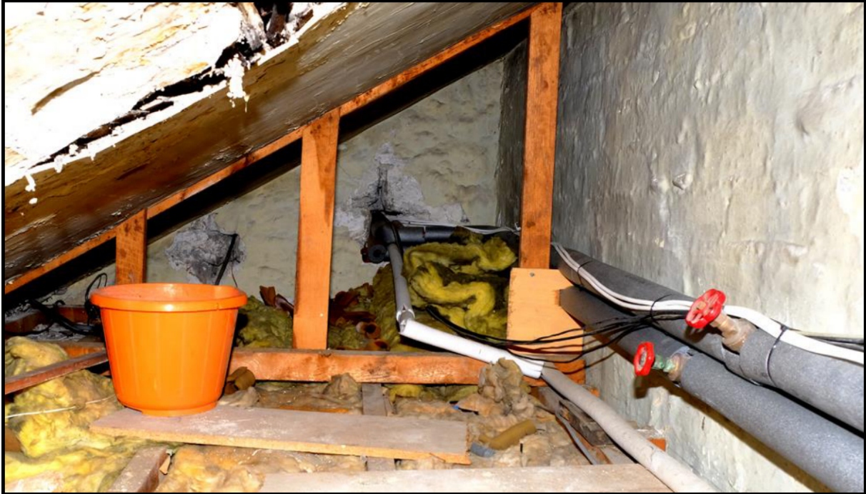
Internal view of roof void above utility room (western end)
