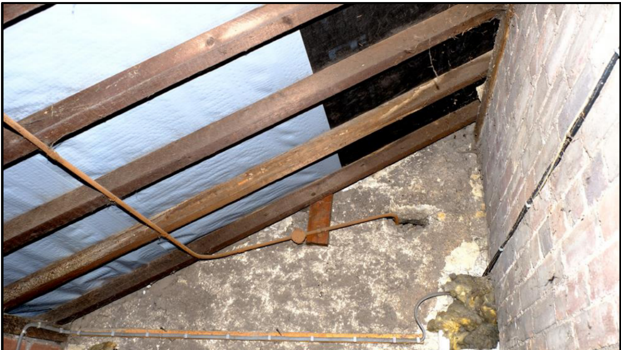
Internal view of roof void above utility room (eastern end)
