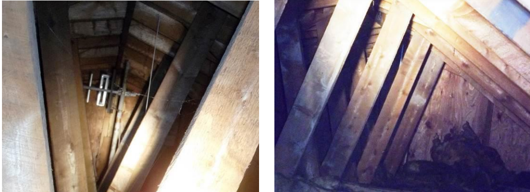
South-western gable end
