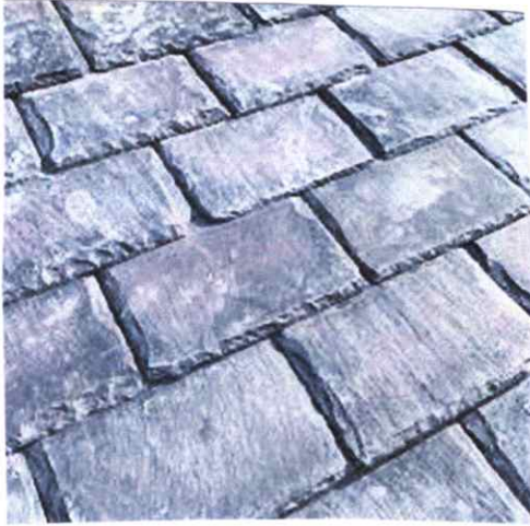
Blue slate roofing
