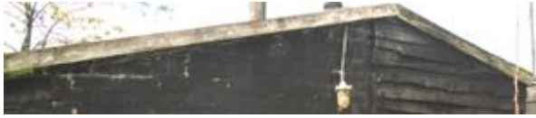
Timber barge boards to gables.
