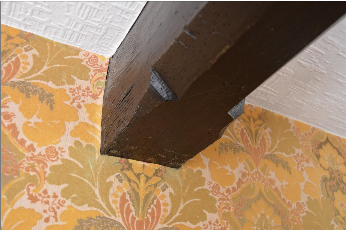
PL07: View of chamfers and moulded stops to a ceiling beam within the ground floor living room.
